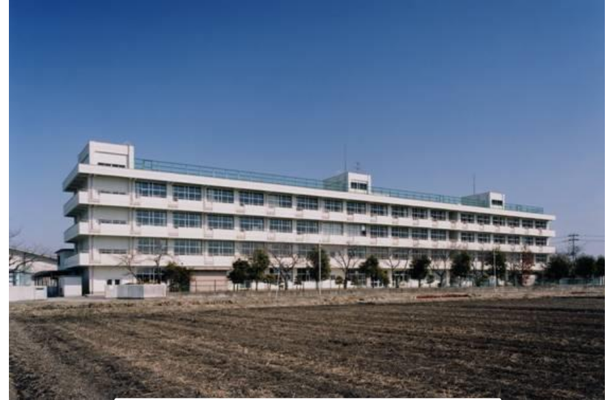
An elementary school that went under additional earthquake-proof work
