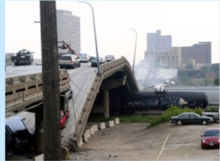
Mississippi River Bridge Collapse in US (2007.8.1)
